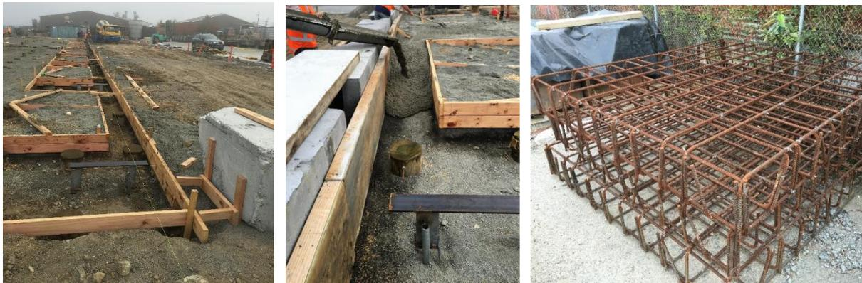
**Figure 12. SFRC Pile caps and capping beams without conventional reinforcement (right photo shows the original designed but since abandoned reinforcing cage).**
