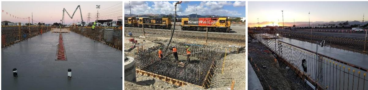
**Figure 13. SFRC and conventional reinforcement for Kiwi Rail Locomotive Wash Raft Slab**
