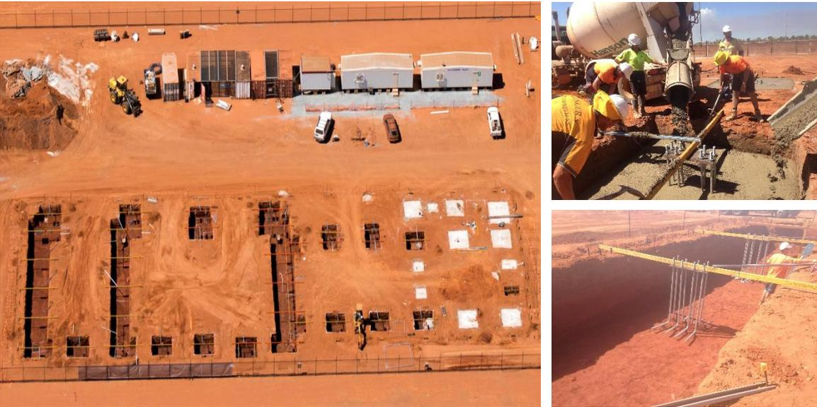
**Figure 10. Komatsu Heavy Machinery Warehouse Foundation reinforced with steel fibre only.**
