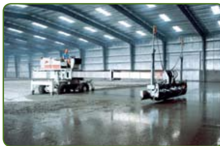
3. In the industrial flooring, steel fibres are a proven and recognized solution. Already more than 1/3 square meters is reinforced with steel fibres.
