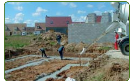
4. Pouring the foundation of a house in steel fibre concrete.
