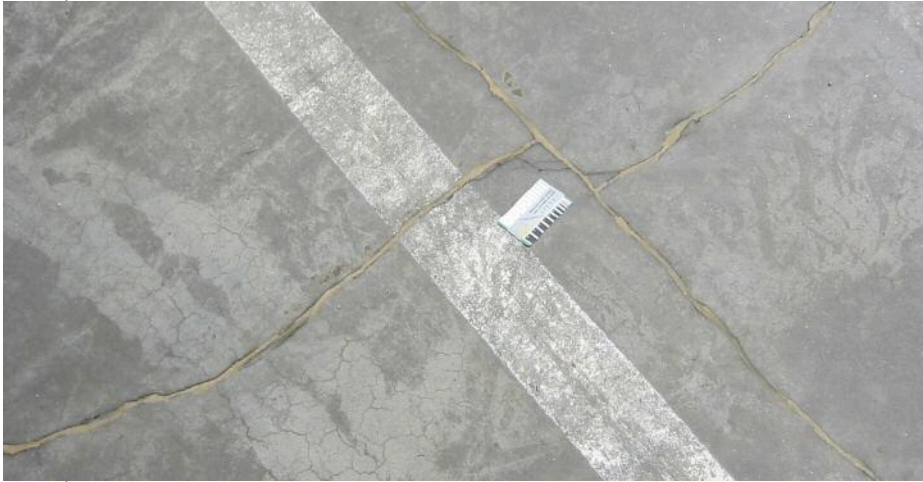
Above: Concrete cracks by shrinkage or loads. Adding steel fibres not only works on temperature and shrinkage control, but increases the load bearing capacity
