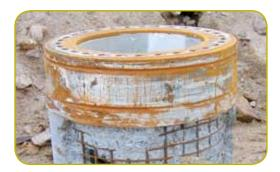
Traditional pile foundations can suffer severe damage in extreme ground conditions
